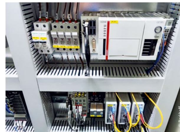
A CX2040 Embedded PC with a quad-core Intel® Core™ i7 processor offers high computing power for controlling the many servo axes in the installation.
