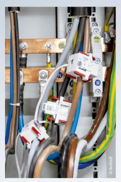
The split-core current transformers of the SCT series facilitate the retrofitting and integration of existing plants and buildings into a comprehensive energy management system.
